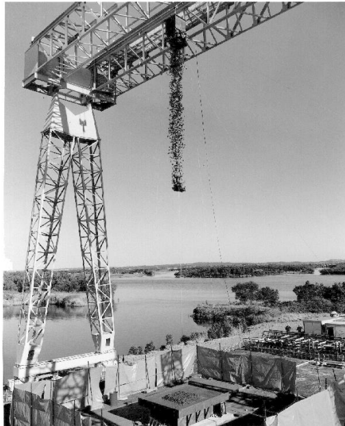
Figure 3. Photograph showing an overview of a drop test in progress. BHP HBI at an equivalent rate of 4000t/hr, from 25 m, onto an existing HBI layer.
